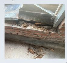
Shows the crumbling windowsill and faulty mortar under the open window space.
