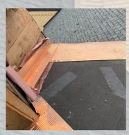
Shows the new wood installed, tarpaper and new copper flashing and paper backing to help with drainage off the deck.
