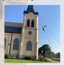
Shows the North Tower, the removed louvers and openings that need repair. The winch cable attached to the truck allows Vasa to raise lumber, tools and materials to their workspace through the windows.
