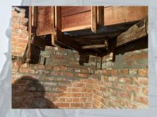
Shows the new mortar and reinstalled bricks (5 or more layers) to support the corner. Also, the cut off vertical support beams that line the interior of the steeple.
