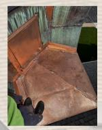
Copper and access hatch soldered and completed.
