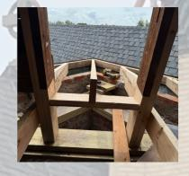
Shows the new horizontal and vertical wood structure that Case is standing on. You can see the pitch to drain the water away from the tower.
